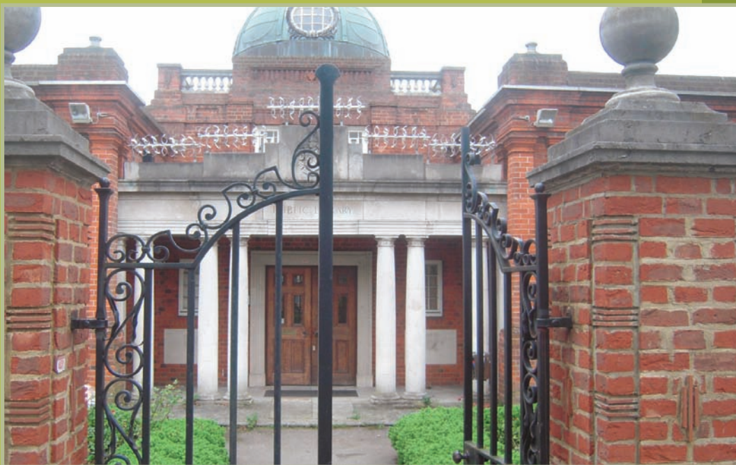
Anti Climb Spikes and Steel gate
