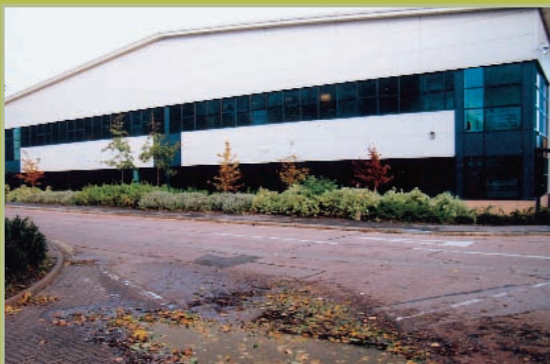
Crime Shield screens installed to commercial unit for glass protection, HS Shoreshield type
