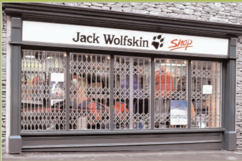
Retail Installation of Sliding Grille type HS1010, non insurance rated type
