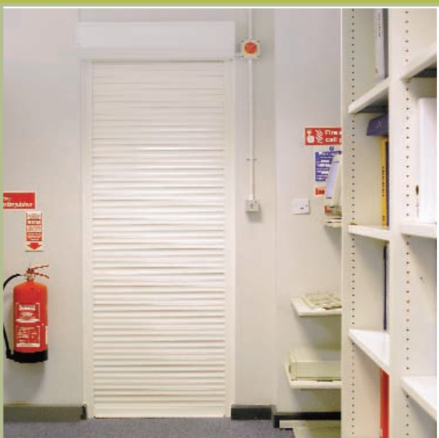
Harling HS Smoke barrier, fire rated curtain partly closed
