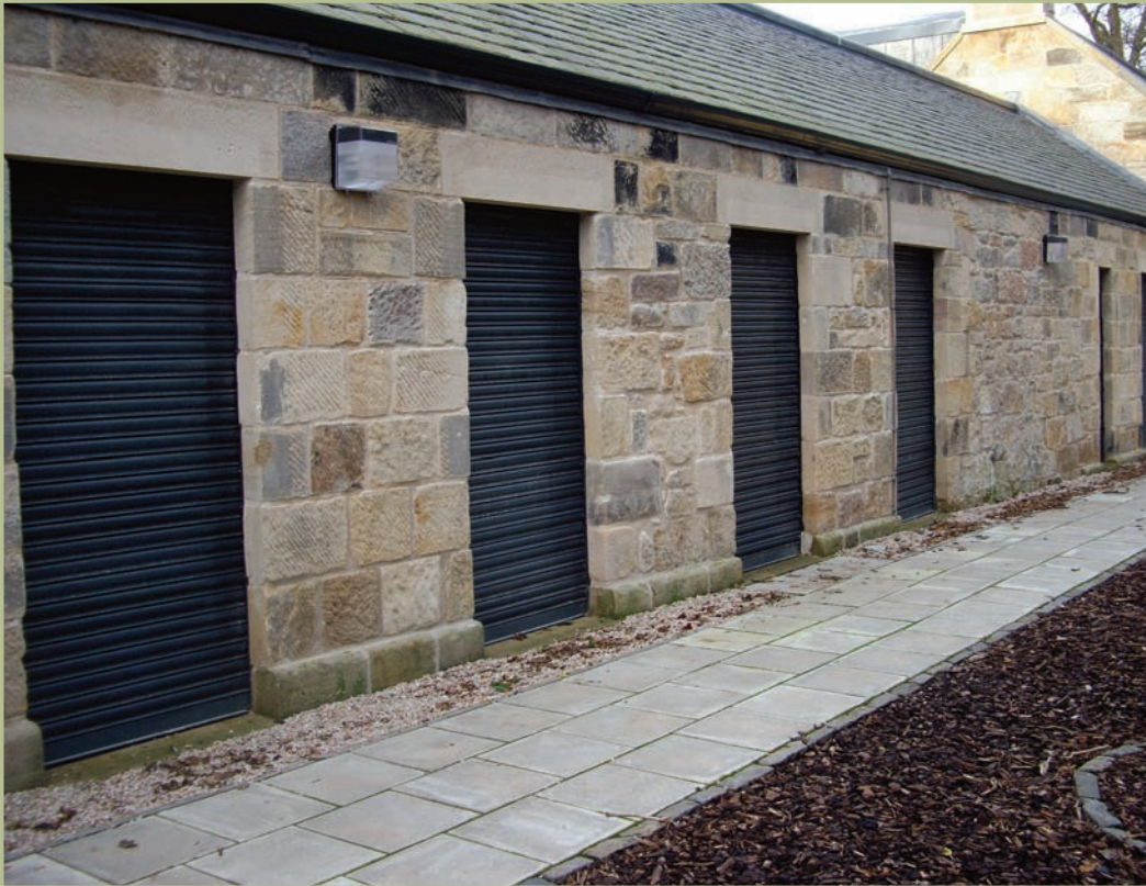
Powdercoated HS75 perforated steel shutters to grade 1 listed building
